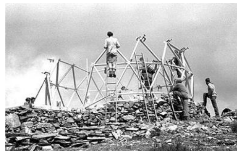
Construction of the MUMC Memorial Hut on Mt Feathertop in 1966
